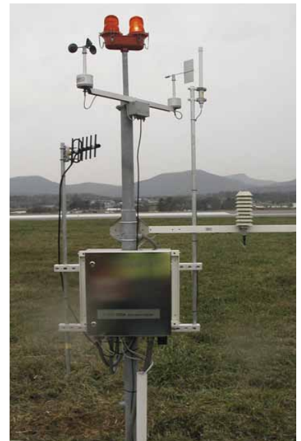
RWIS installed on a Runway – RPU with sensor suite (atmospherics)
